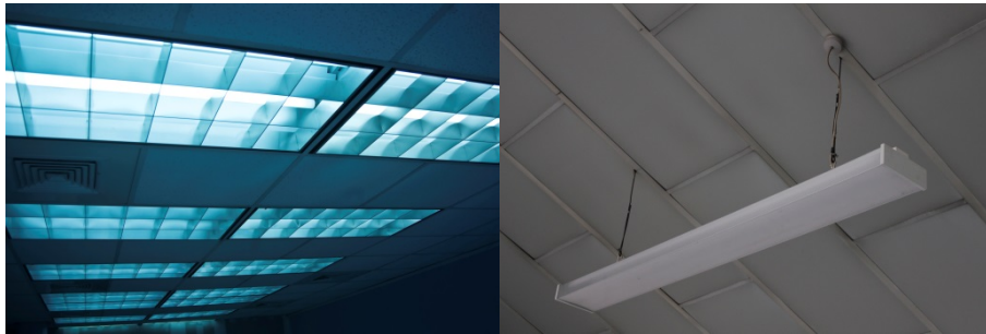
Figure 28: Recessed troffers with louvres to direct light output (left) and a pendant batten with diffuser (right)
