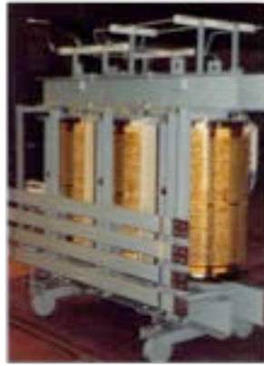
(b) 750kVA dry type: open winding
